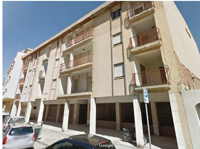
Fig. 6: Front view of the council housing building
