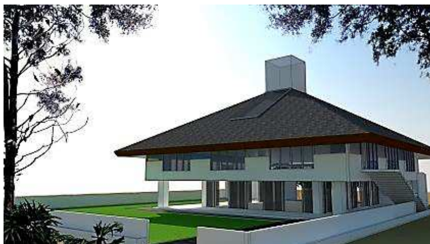
Fig. 8: 3D illustrations and photos of the Eco Pesantren mosque showing openings at the side of the building
